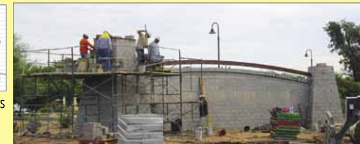
Construction as of August 4, 2016.
